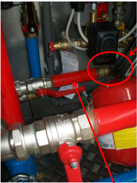
Curva 90° MF 1" 1/4 Nipples 1" 1/4 Curva FF 1" 1/4
